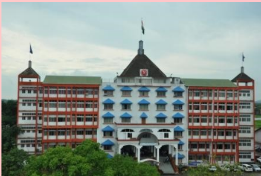
Front view of GIMT building
