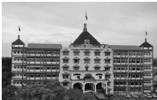
Front view of GIMT building
